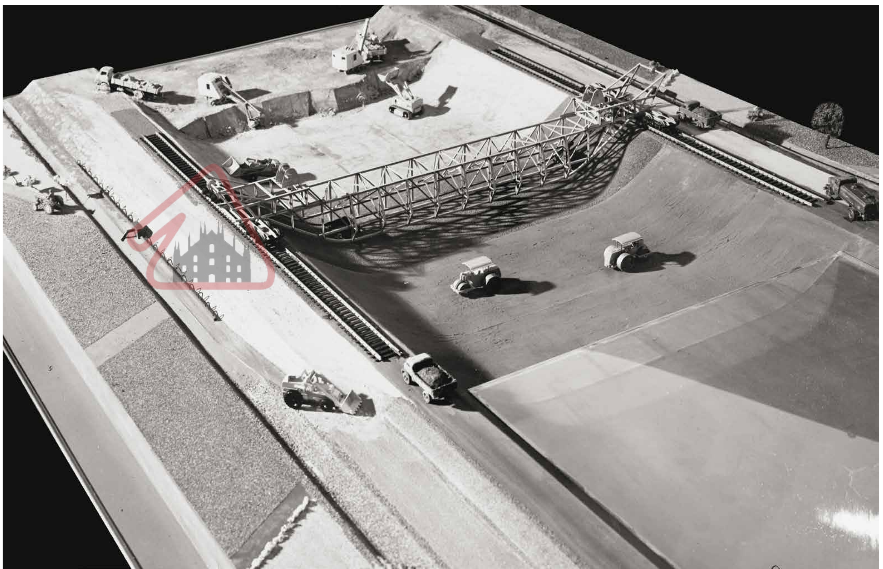
Plastic model of the profiling and waterproofing work site for the first stretch of the canal, between Cremona and Spinadesco, author unknown, 1966, silver salt print (180x210 mm). ASM, Fondo Consorzio del Canale Milano-Cremona-Po.
